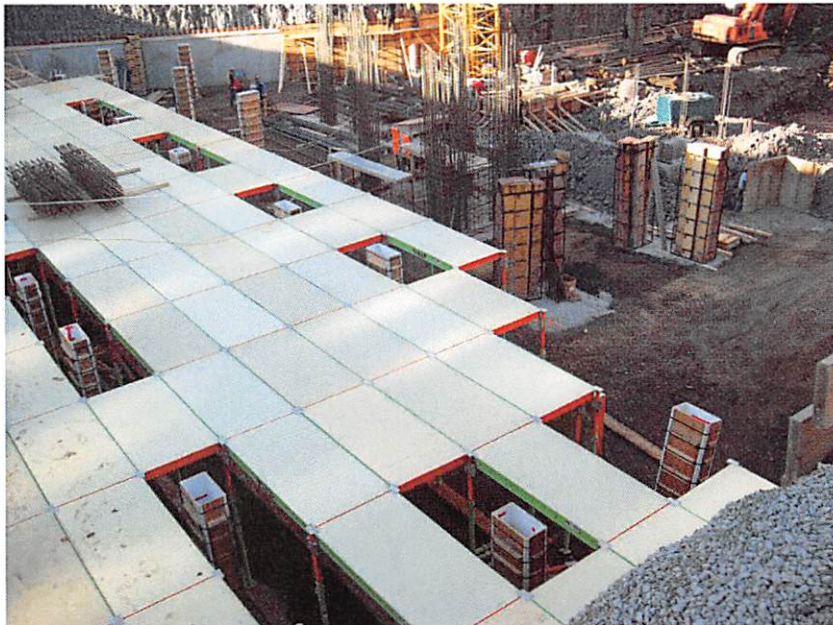
Method #2: Rebar can be dropped in from the floor above and the tie can be viewed from an inspection window cut into the column.
